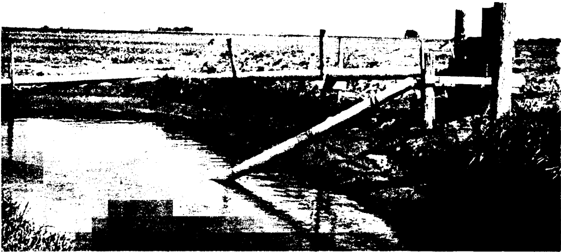
Figure 2. A dugout with a centrifugal reuse pumping plant. Runoff water being pumped back into the same field.
