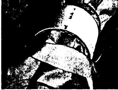
Fig 3 Interior membrane of a tube connected to that of a coupler with a Velcro fabric fastener.
