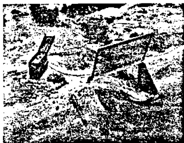
Fig. 3. Drop-closed gate in a ditch turnout to a level basin.
