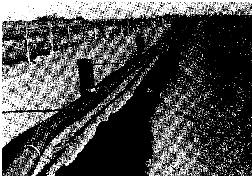
Figure 4. An assembled buried-pipe runoff control system ready for installation.
