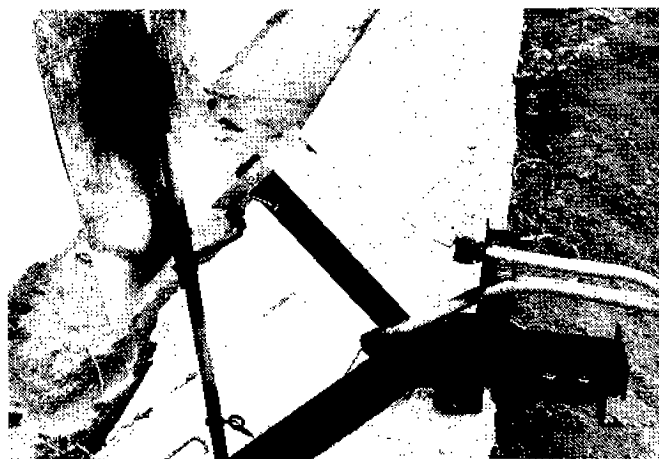
Figure 15—Photo of a drop-closed gate for a pipe turnout showing the mounting bracket, gate latch, and trip-cord release.
