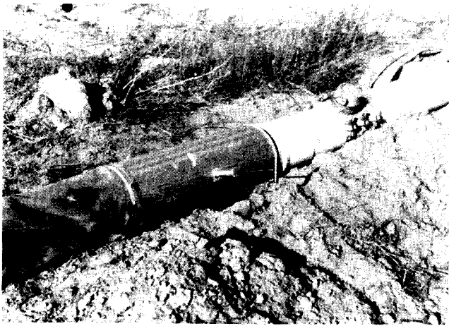
Figure 8—Photo of manual valve with a pull-push handle to change irrigation sets.
