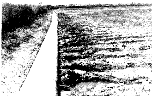
Figure 2—Photo of 300 mm (12 in.) diameter dual-conduit tubing in the distribution mode. The tubing replaced siphon tubes and the ditch seen on the left.
