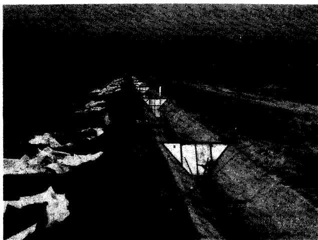
Figure 7—View of a semi-automated border irrigation system using center-of-pressure check gates.
