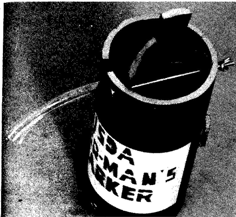
Once you have things as you want them, it is time to cut the holes that will allow attachment of the unit to the spray boom. Cut two D-shaped holes, as shown in the drawings, so there is a 1-inch band left for the attachment. Take the 1-inch wide reinforcing strip you cut and glue it on top of this strip, to make it stronger. The common types of "super glue" work fine for this gluing task.
