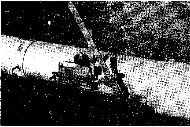
FIG. 4 Semiautomatic irrigation valve with a modified trip linkage for safe operation.
