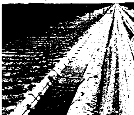
Fig. 1 Automatic cutback furrow irrigation system in concrete-lined ditch
