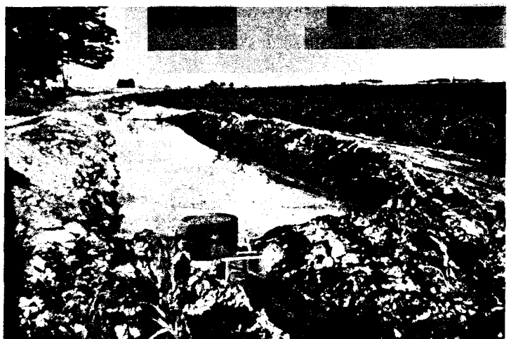
Fig. 6. This sediment basin is nearly full after collecting sediment from the tailwater from a 5-acre corn field.
