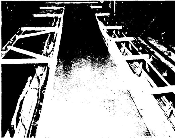
FIGURE 25.—Rectangular channel C. The boundary was troweled to produce the smoothest surface possible.
