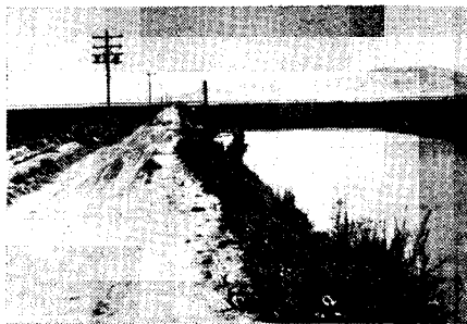
FIG. 1 Sequence-type return system with reservoir, pump and short return pipe. Stored water collected from an upper field is used as a separate supply and is pumped across the road to lower lying field.
